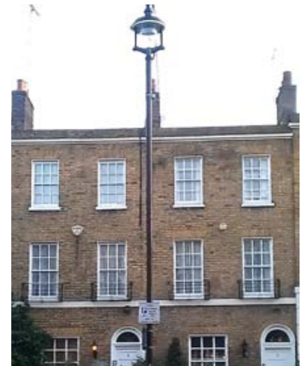
Traditional Street Lighting
